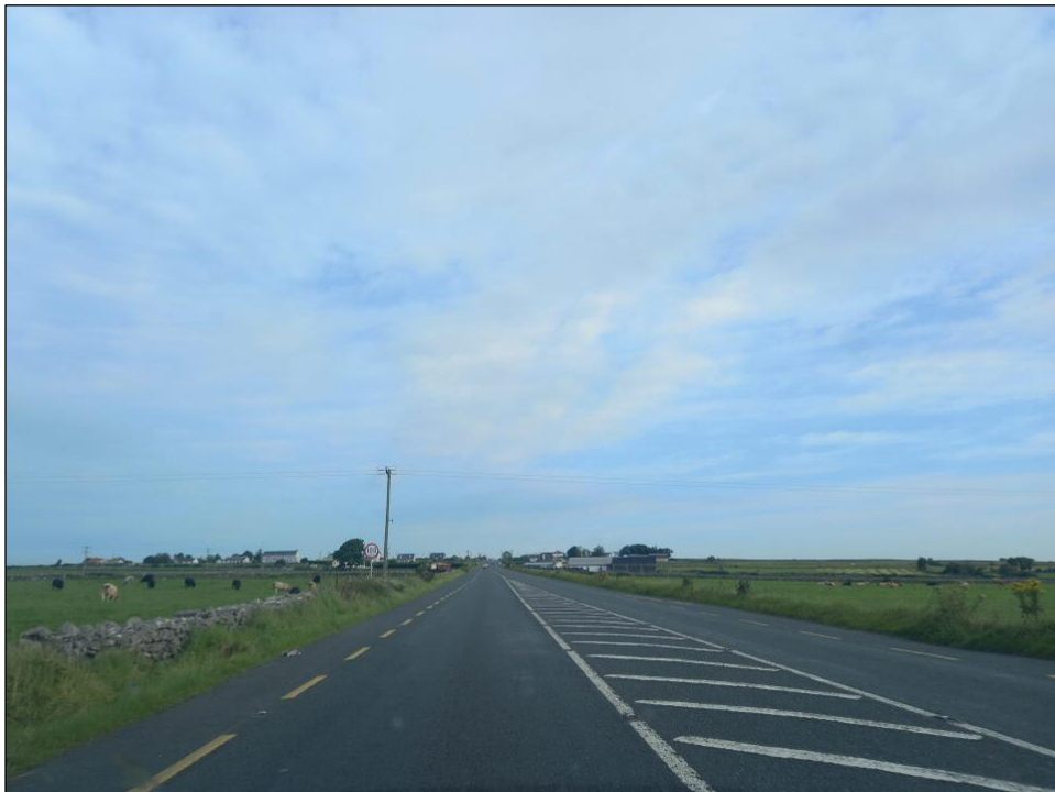
Plate 6-16 The Proposed Grid Connection underground cabling route as it leaves the Proposed Wind Farm site along the N83
