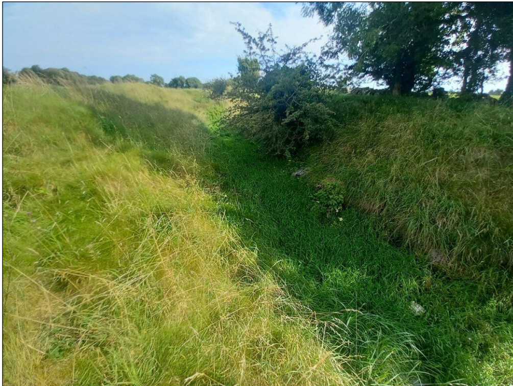
Plate 6-18 Water crossing 1 along the Glennafosha River
