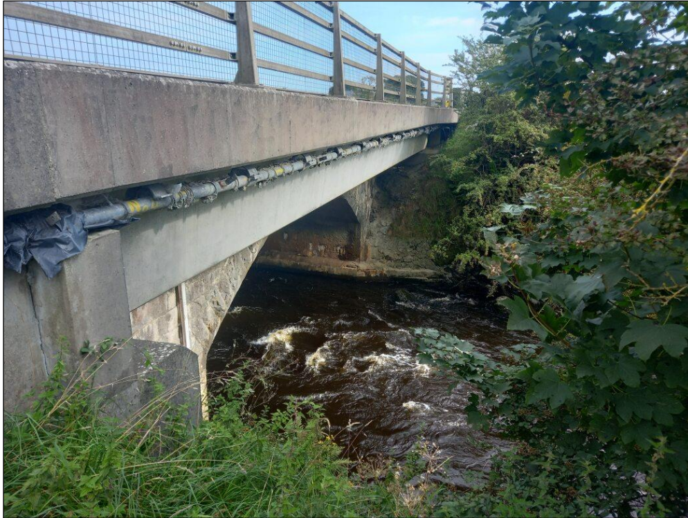
Plate 6-19 Water Crossing 2 over the Clare River
